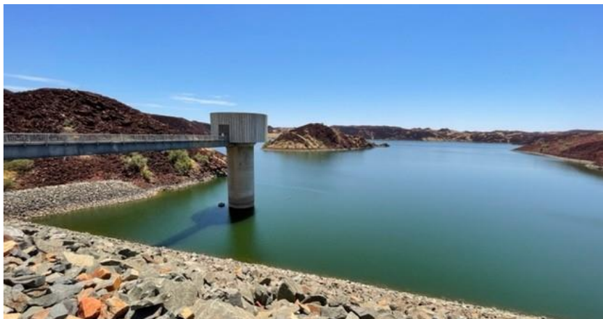
Figure 3: Harding Dam, West Pilbara
